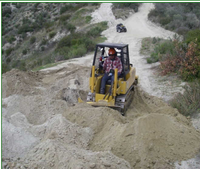
Above: Chunking with an excavator along a dozer line. After chunking, then the equipment spread topsoil and slash from the dozer piles over the treated area.
